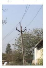
**Limitations of the present system:** As per our field experience, we are facing many issue for tilting of V Cross or top fitting due to that the clearance between the conductors reduce and chances of faults are increase. And also which is esthetically not look good.
